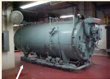
**Fire Tube Dry Back Boiler**
