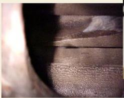
Accumulated sludge from lack of blow down formed on top
