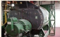
**Fire Tube Wet Back Boiler**
